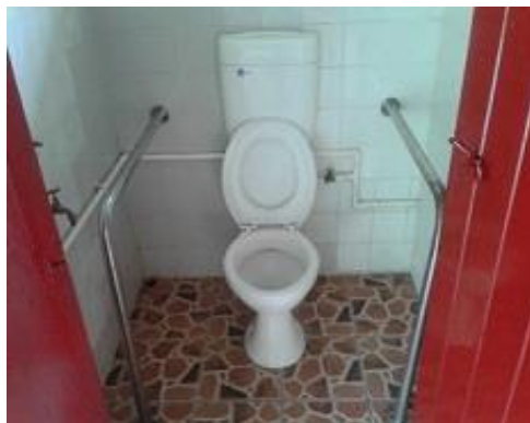
Accessible toilet at Bayly Memorial School in Ra
